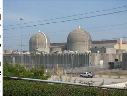
Units 1 and 2 at Plant Vogtle Nuclear Power Plant near Waynesboro, Georgia
