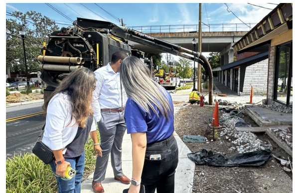
PSC Gas Staffers watch the Mud Dog 1200 Vacuum Excavator in action
